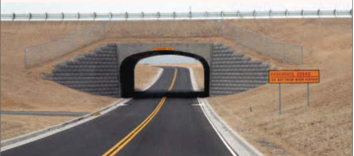
On the other side of this overpass is the ride and handling track, which has intentional defects ranging from mildly annoying tar strips and short waves to multiple waddles and deep troughs that bounce the stomach into the throat. The overpass is one of two circular tracks that simulate freeway driving. (U.S. Army photo by Mark Schauer.)
