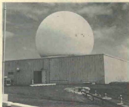
Ascension Island dome-enclosed radar.
