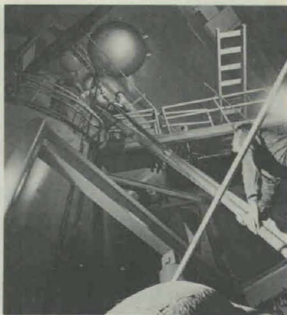
Army Nuclear Power Field Office power reactor, Fort Belvoir, Va., is stationary but components are transportable by air for remote installation. It set stage for first portable nuclear plant at Camp Century, Greenland.
