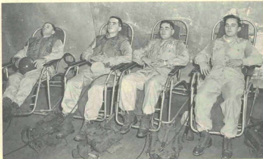
With bodies wired to record skin temperatures, participants in tests of experimental hot-dry (desert) uniforms, relax in tropic wind climatic chamber.
