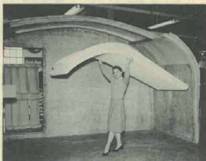
Plastic foam wall section is light enough to be carried easily by girl.
