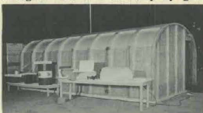
Completed plastic structure, 24 feet long by 16 wide, stands behind its compactly packaged building components (on table at left) and model of its shape and reinforcement structure.
