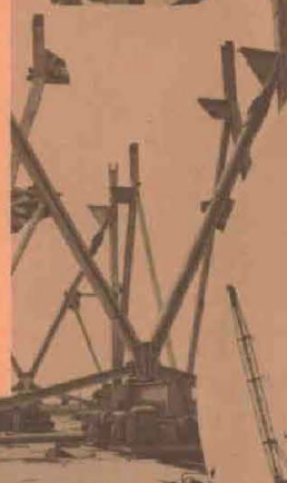
GIRDERS RISE SKYWARD
