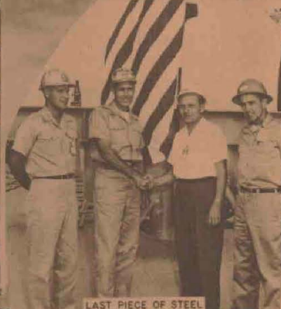
LAST PIECE OF STEEL
