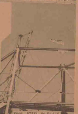
FINAL STEEL IN PLACE
