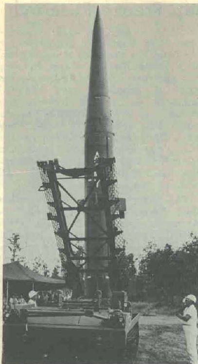
Army's PERSHING missile erected on its mobile transporter-launcher.
