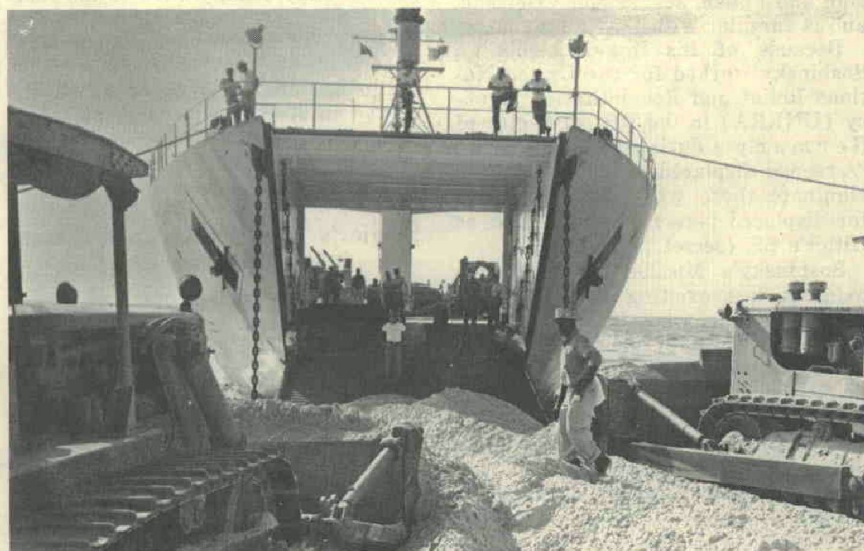
Bulldozers push sand near ramp of USS PAGE in preparation for laying of track and unloading of gun tubes onto the beach at Barbados, W.I.F.
