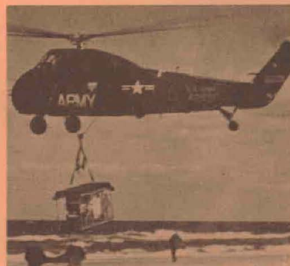
Helicopter air-lifts distillation unit from trailer to field operation site.
