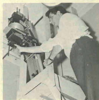
Robert M. Petty, Adjustments and Test Branch, operates precision condenser enlarger to provide photographs used in producing lunar maps.
