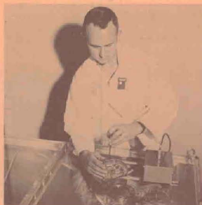
Physicist Richard Dysart adjusts missile component for testing on Pulsed Neutron Generator in Nuclear Effects Lab at White Sands, N. Mex.
