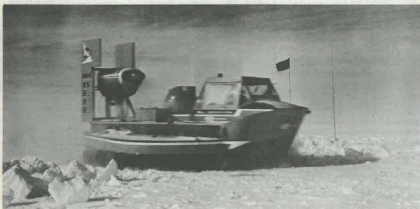
CARABAO crosses simulated 4-foot-wide crevasse during recent tests.
