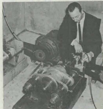
PROPULSION TEST unit chief Ralph Vecchio adjusts gauge of a spin test stand developed at Picatinny Arsenal for 105-155mm. rockets.
