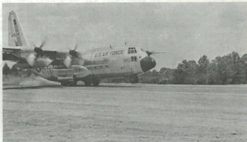
U.S. Air Force C-130 (Hercules) "touches down" successfully on the completed runway during tests conducted at Fort Lee, Va. The runway was constructed entirely of the experimental airfield membrane which is fabricated from nylon.
