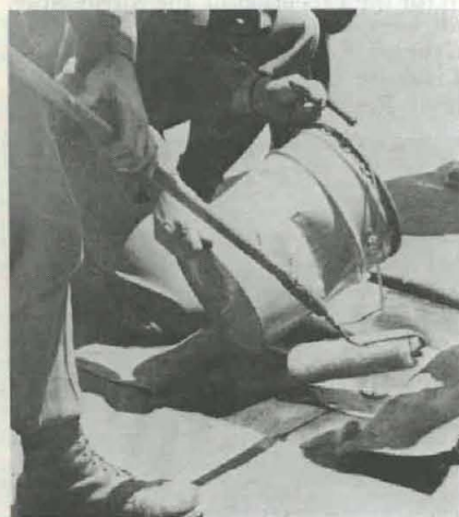
Should damage occur during operations, repairs are simple. A patch is cut from the spare membrane panel and cemented under the damaged area.
