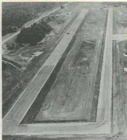
Neoprene-coated nylon membrane simplifies construction of a complete assault airfield after the site has been cleared, graded and compacted.
