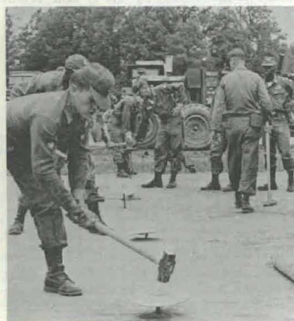
Panels are anchored to the ground with steel "tacks." Edges are then reinforced with two layers of membrane surfacing and cemented in place.
