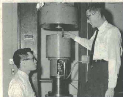
WATERVLIET ARSENAL researchers Dr. James Uy and Charles Nolan are shown with the press of their own design in which they have successfully extruded high-strength, lightweight alloys similar to that held by Nolan.
