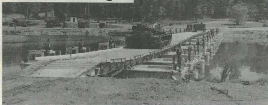
TWELVE MAB units provide 334-foot bridge span for river crossing.
