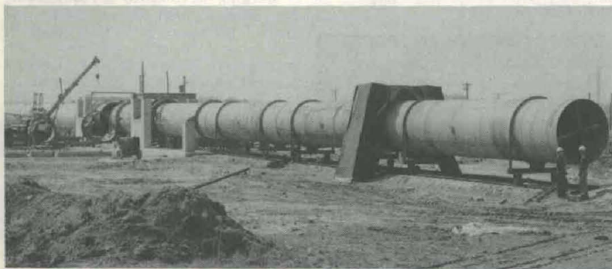
SHOCK TUBE facility nears completion at Army Ballistic Laboratories, Aberdeen (Md.) Proving Ground. It will be used to study simulated nuclear-blast effects on air-breathing engines of Sentinel System antiballistic missile defense.
