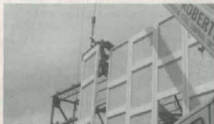
"PANELISTS" prepare to "seat" a decorative concrete panel as a mobile crane swings it into place on framework of Joint Command Headquarters building at Aberdeen Proving Ground.
