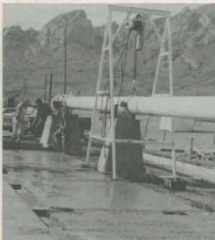
FOUNDATION is set for a galvanized iron shelter to house the absorption cell and the environmental controls.
