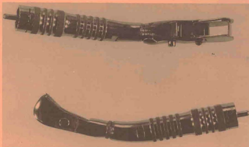
MUCOSATOME blade is manufactured in two widths, 4mm and 2mm, pictured above in two views. The U-shaped blade (at right end, top view) reaches out beyond the guards on either side and makes a short stroke forward. The attachment pin (left end, top view) connects to a standard dental handpiece.
