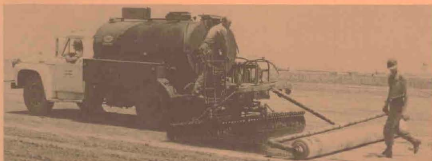
CE construction engineers lay polypropylene cover over prepared subgrade.
