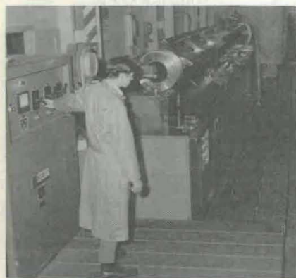
MATERIALS TESTER Donald W. Horton starts a 175mm gun tube turning as a fellow employee (under canopy at rear) makes his way forward along the tube with a black light scope. The process is part of the Aberdeen Proving Ground Material Evaluation Unit's mission of inspecting each weapon before it enters the Army inventory.
