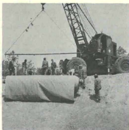
A 25,000-barrel hasty storage fuel reservoir is placed in position on the revetment by a 20-ton rough-terrain crane equipped with spreader bar.
