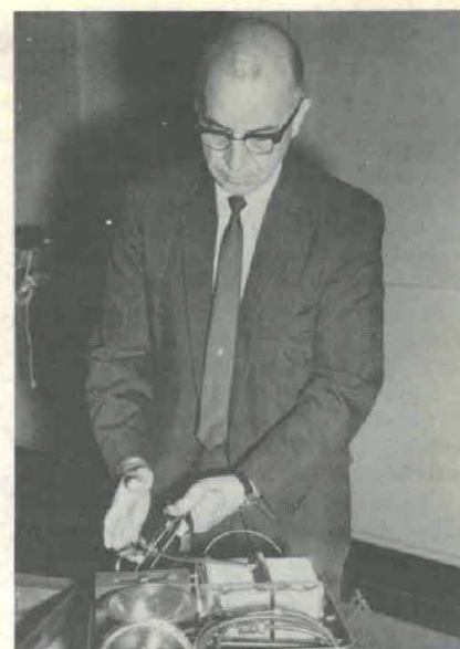
MERDL Technical Director Benjamin Pile packs 17-pound portable field surgery lamp into case. Pile developed the battery-powered lamp that can give light eight hours continuously.
