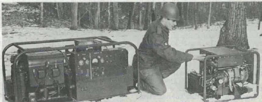
FAMILY OF TURBO-ALTERNATORS is being developed at MERDC to cut costs and ease logistical problems involved in generating electric power in the field. The 10-kw unit shown here is one-fifth as big and weighs 725 pounds less than the standard Army 10-kw engine generator it is designed to replace.
