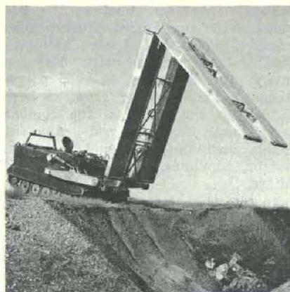
**ASSAULT BRIDGE** is hydraulically launched in less than two minutes by M113 armored personnel carrier. Constructed of a stress-carrying composite of extruded aluminum, the 33-foot-long, 2,700-pound bridge supports 15 tons.
