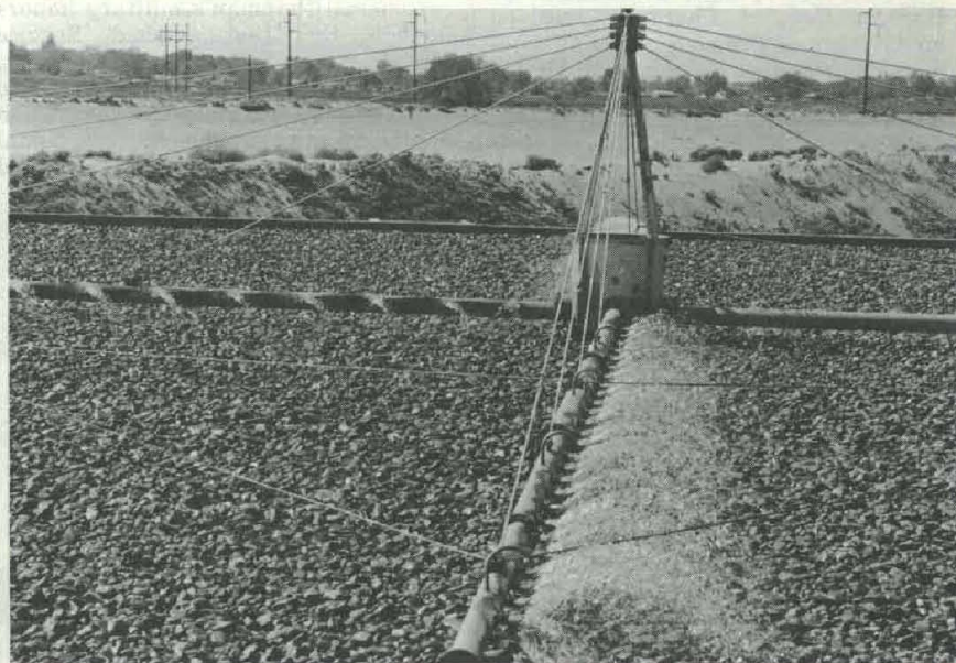
Fig. 1. Trickling filter bed. Note droplet formation along the boom.
