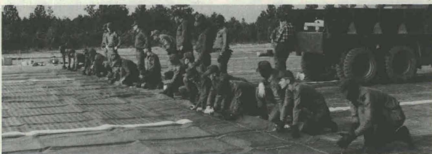
TROOPS from Company "C" of the 4th Combat Engineer Battalion (Airborne), Fort Bragg, N.C., perform finishing touches to a 3,700-foot runway covered with a new heavy-duty, airfield membrane material developed by the U.S. Army.
