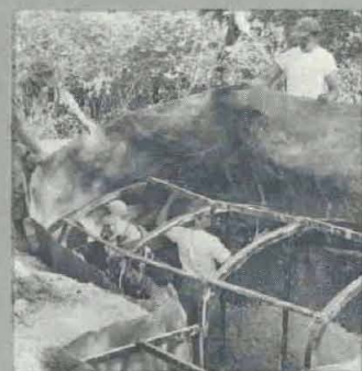
SOLDIERS from the 17th Engineering Battalion, 2d Armored Division stretch a wire-reinforced fabric over the metal frame of an underground bunker in MASSTER (Modern Army Selected Systems Test, Evaluation, Review).
