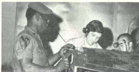
ARMY and civilian mechanics work together to rewire the weapons system in the wing of a Cobra helicopter gunship in preparation for evaluation by MASS-TER.
