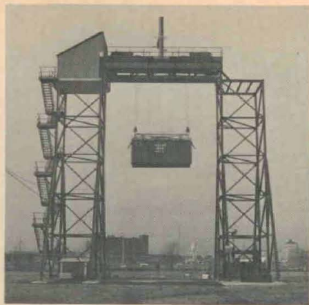
INTEGRATED Test Rig for the HLH Cargo Handling System simulates operational cargo lift cycles with a MILVAN container and an automatic load device.
