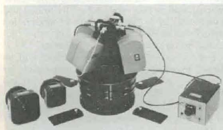
Fig. 1. Single-Lens Multiband Camera
