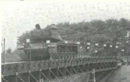
M-60 Tank Crosses Medium Girder Bridge
