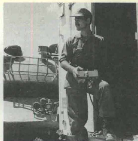
TONE IMPULSE device is operated by SGT Marvin Duhr for remote guidance on an M-47 used for target tests at WSMR.
