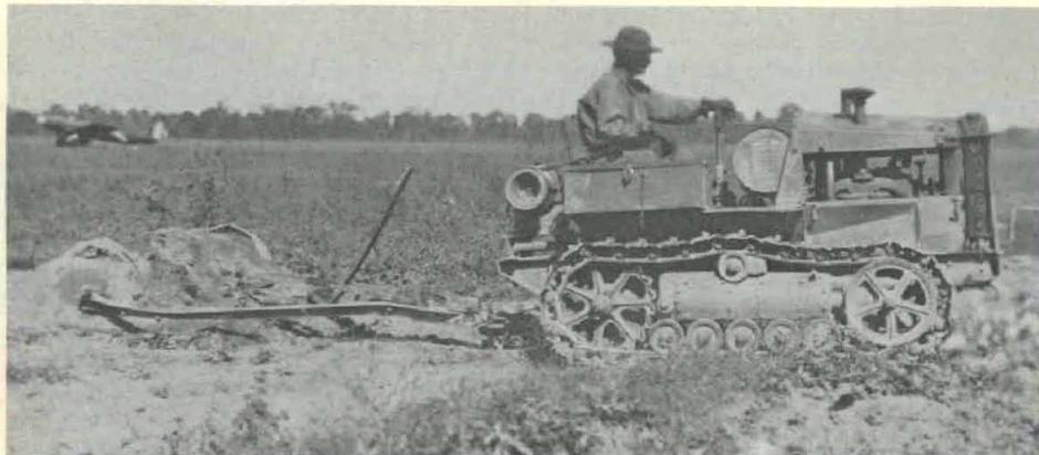
TRACTOR MOBILITY has come a long way since this 1935 CLETRAC 3-ton tractor with towed roll-over type scraper.
