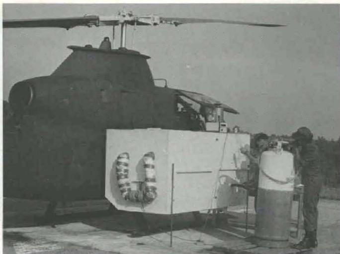
**REFRIGERATION UNIT** devised by USAADTA personnel to meet requirements of the Prototype Qualification Test-Contractor, to verify test criteria under a very tight test schedule, coupled with an austere test budget.
