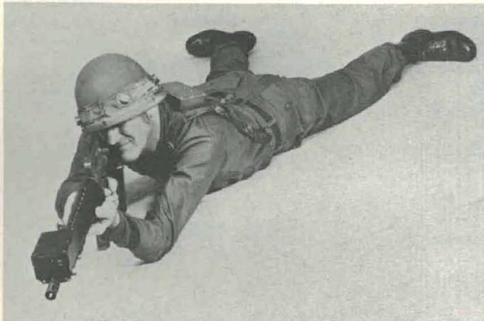
MILES system for M16 rifle. A buzzer indicated kills or near misses when the laser beam strikes detectors on the soldier's helmet or torso harness. To silence the buzzer, the soldier removes a key from the transmitter of his rifle and inserts it into his harness, which, in turn, disables his transmitter.
