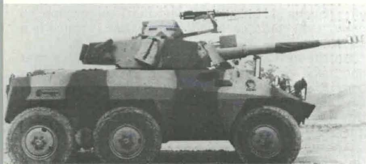
Brazilian EE-9, Cascavel 90mm gun, 6x6, armored recon vehicle, used in Latin American and the Mid-East (1975).
