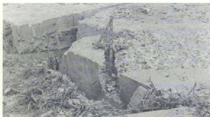
Side view of cut made by water jet demonstrated by University of Missouri. Also note surface concrete (at right of photo) that was removed with only a few passes of the water jet.
