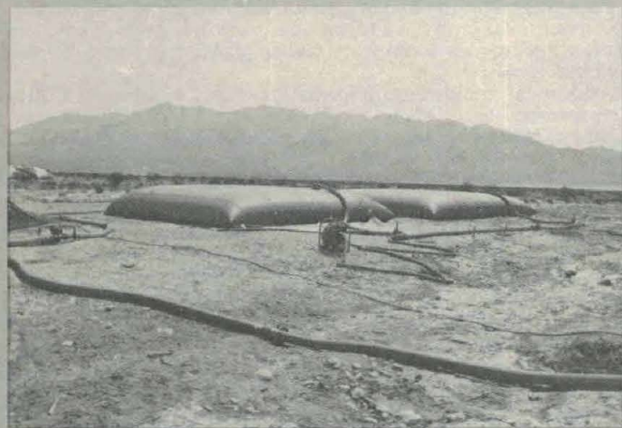
These 20,000-gallon tanks will become part of a field water supply system for the Army and Marines.
