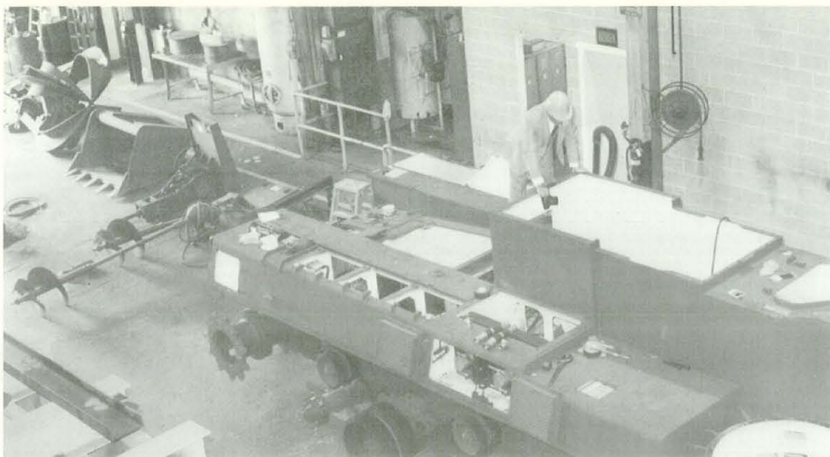
A weapons system staff manager looks into the crew compartment of a test bed. The circular area to the bottom right is the mount for one of its two telescopic arms. Behind the test bed to the upper left are various arm attachments.
