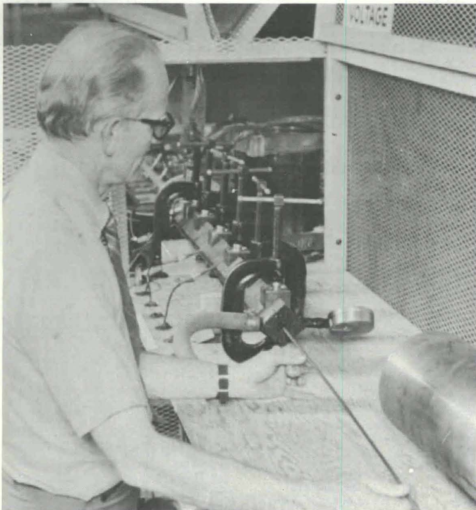
Awardee Henry Burden operates small rail gun used for experiments to determine properties of an arc armature. Electro-magnetic guns may be used where very high projectile velocities are required, such as in air defense or outer space applications.
