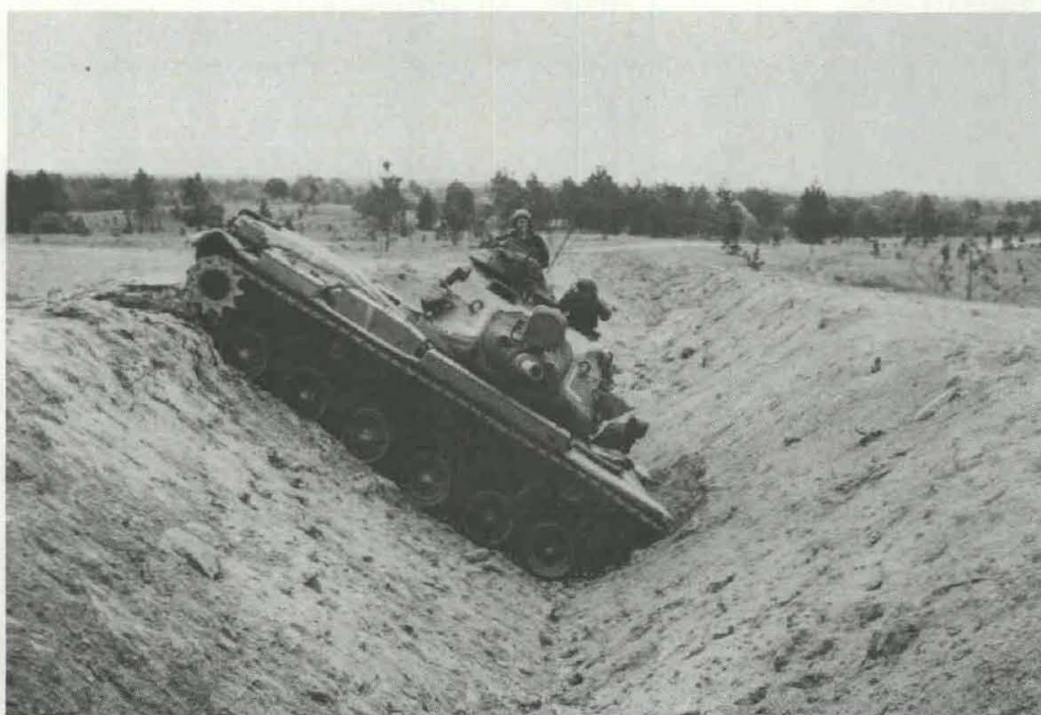
Cross-section of anti-tank ditch created with buried plastic pipe at Ft. Polk, LA.
