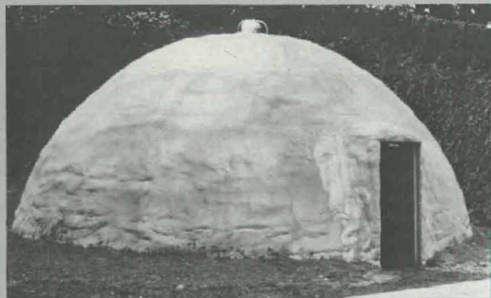
A 28-foot USA-CERL foam dome constructed during a mobilization exercise at Fort McPherson, GA, in 1982.
