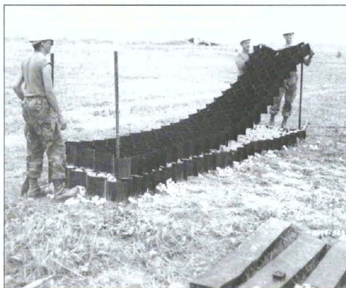
Soldiers from the 52nd Engineer Battalion at Fort Carson, CO, expand and fill sand-grid sections with gravel for a live-fire test with light anti-tank weapons. Layers of sand-grid are stacked and filled to form a protective revetment. Collapsed sections of sand-grid are shown in the lower right.
