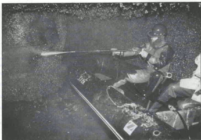
Removal of zebra mussels from Detroit Edison's Monroe Power Station using high pressure water.
