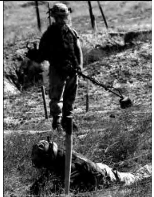
Combat engineers from the Army's 10th Mountain Division (Light) (10th Mtn Div (L)) work in teams of two while clearing mine fields at Bagram Air Base, Afghanistan. One Soldier initially probes the area, and the other Soldier sweeps it with an AN/PSS-14. (U.S. Army photo by SGT Greg Heath, 4th Public Affairs Detachment (PAD).)
