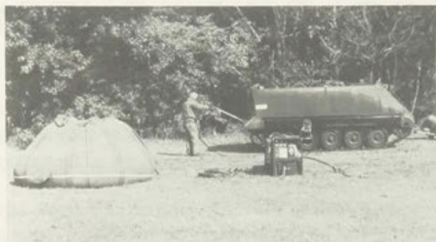
LIGHTWEIGHT DECONTAMINATION SYSTEM DECONTAMINATING A M113 ARMORED PERSONNEL CARRIER
